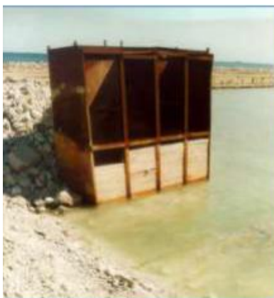
Figure 10.10 Weir box and cross section of Weir box
