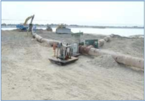
Figure 10.8 Splitting of shore pipeline to different areas
