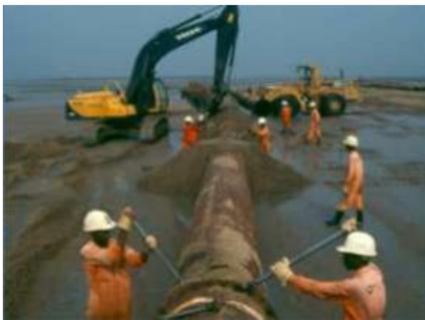
Figure 10.9 Extension of pipeline at reclamation area
