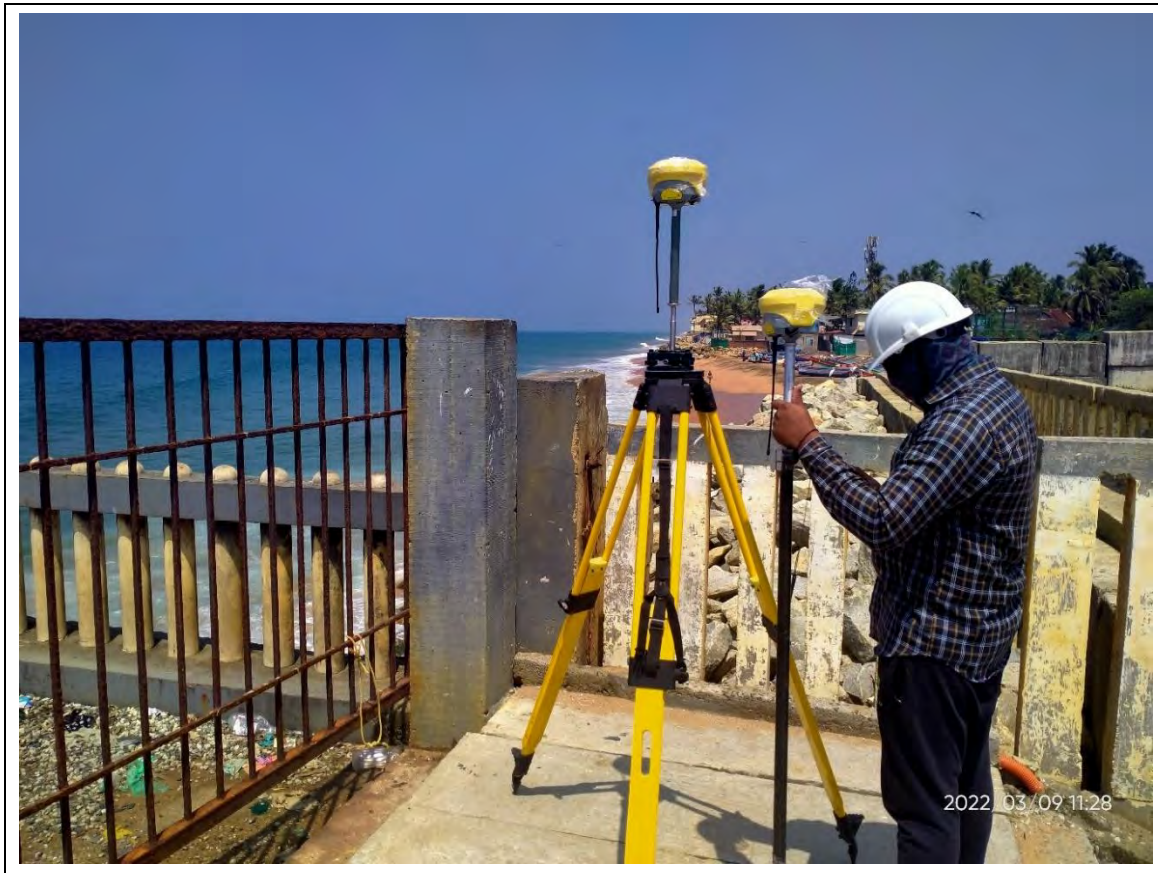
Figure 5-8: RTK System with base station and rover
