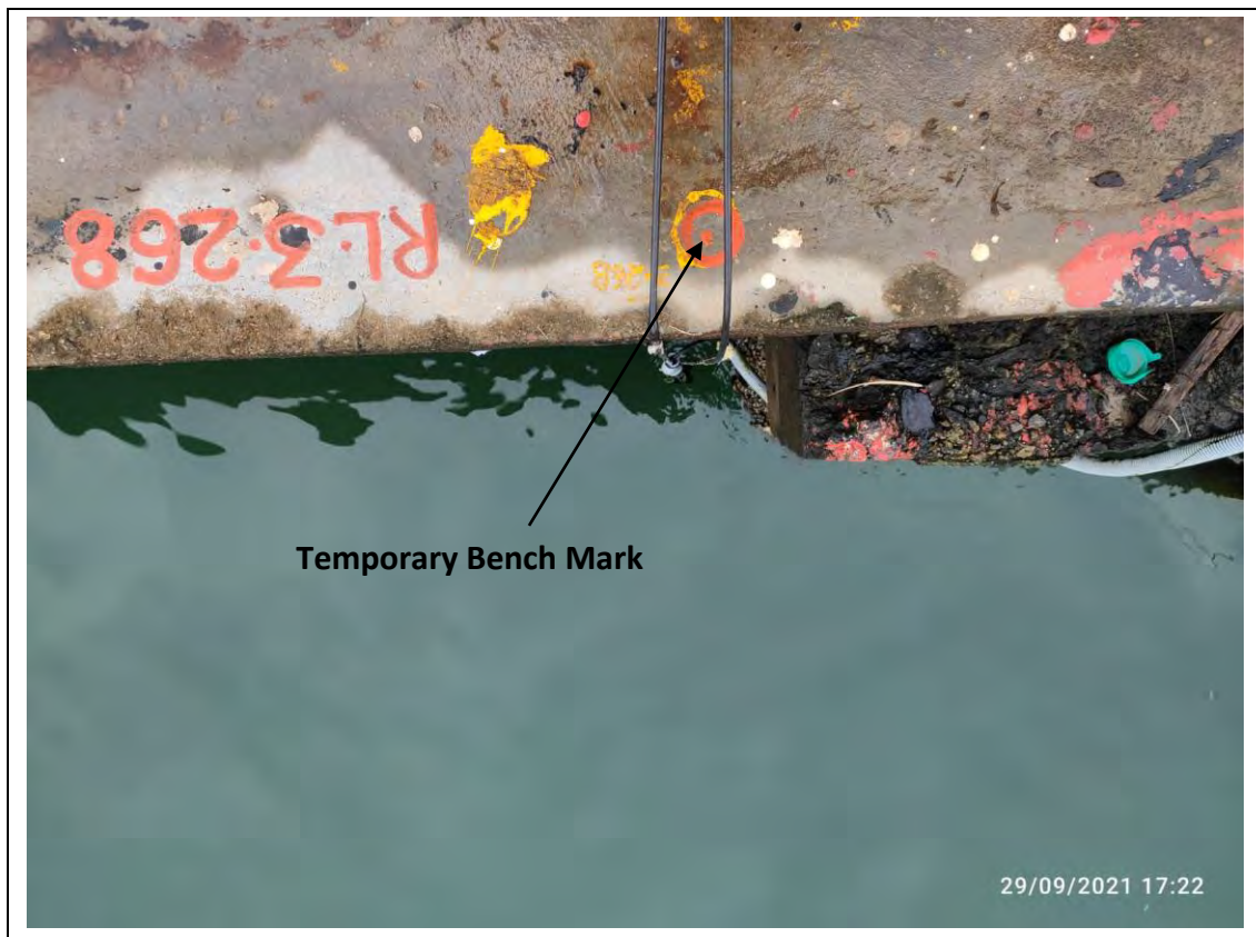
Figure 6-1: Location of TBM
