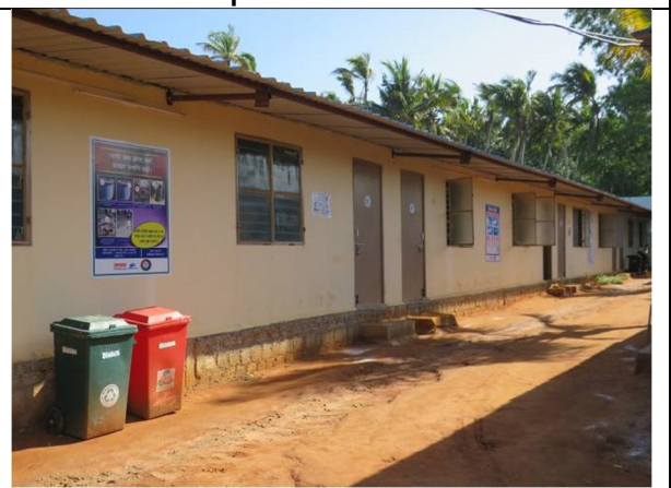
COLOUR CODED DUST BINS INSIDE THE CAMP of M/s AFCONS
